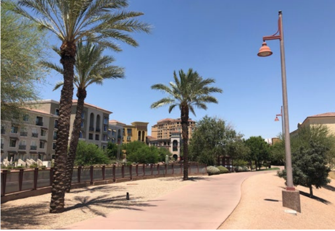
Gravel area between pedestrian path and railing, facing east.
