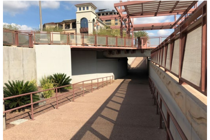
Underpass, facing east.
