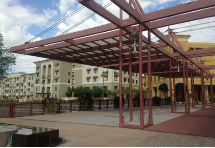
West side of the bridge, facing northwest.
