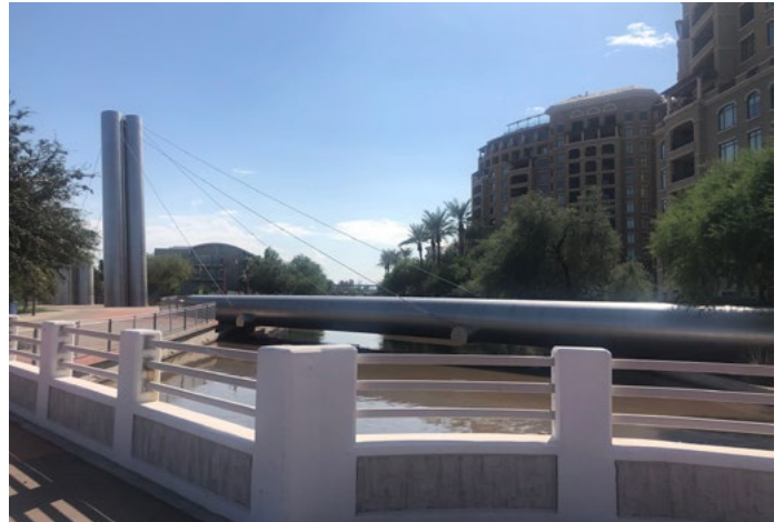
Small canal section east of Soleri Bridge, facing north.
