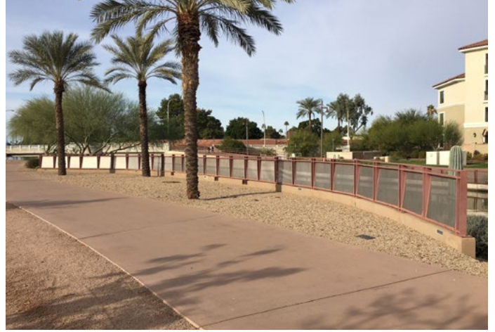
Gravel area between pedestrian path and railing, facing west toward Goldwater Bridge.
