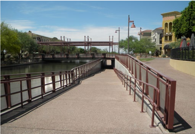
Path and underpass, facing west.
